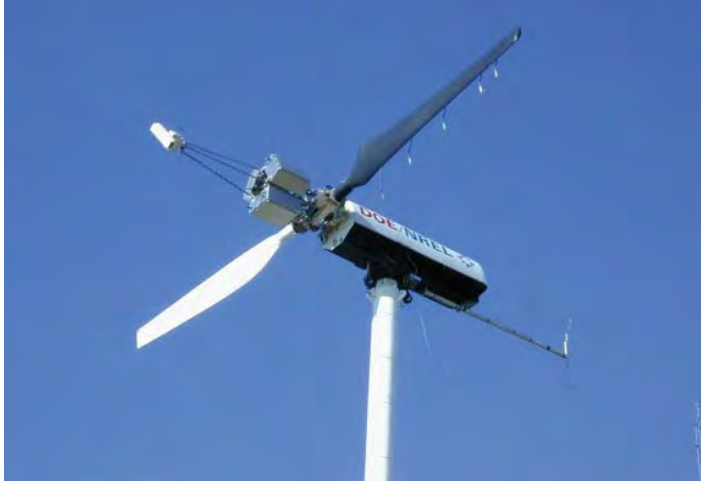
Figure 1: The NREL 10m research wind turbine
